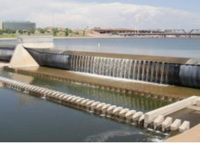
**b.** These can be deflated when pressure is released and hence, even the crest level can be controlled to some extent. Surplus waters would simply overflow the inflated shell. They need extreme care in design and erection and are limited to small projects.
