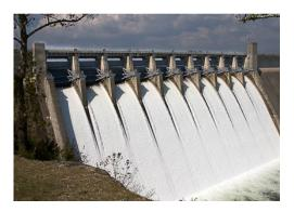
This is the normal reservoir level. If a flood enters the reservoir at this time, the water level will start going up and simultaneously water will start flowing out through the spillway. The rise in water level in the reservoir will continue for some time and so will the discharge over the spillway. After reaching a maximum, the reservoir level will come down and eventually come back to the normal reservoir level.
